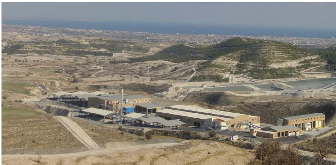
Figure 1: Integrated Waste Management Facility at Nafkias, Kochi Community, Region of Larnaca CYPRUS
